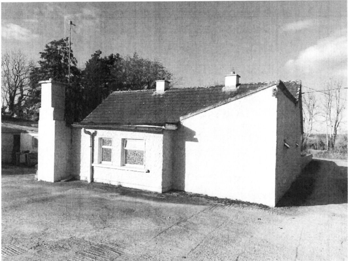
Fig 02. Existing rear extension (1961) to be replaced -
